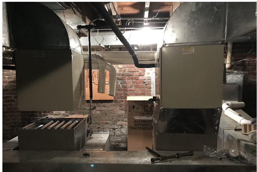
Glenn Riddle from Riddle Repair has started the process of replacing the air conditioning units damaged by the flood waters.
