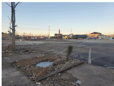
The site of First Presbyterian Church Mayfield's former building was for the most part cleared a month after a tornado destroyed the structure.
